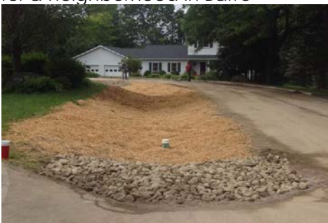
New bioretention facility in Williston
