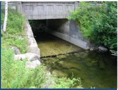
Fixing the non-fish friendly culvert (left), required creating a downstream natural rock weir (center) that resulted in a 'back watered' culvert (right). Doing this did not appreciably reduce flow capacity. This project, completed on Great Brook in Plainfield in 2010, held up through the May 2011 flood and Tropical Storm Irene.
