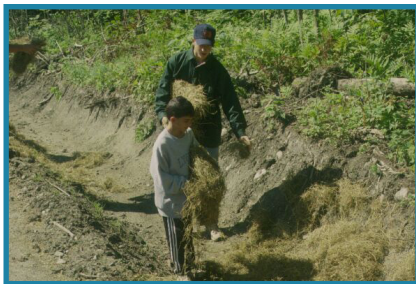
At left, lake association members seed and mulch a newly cleaned ditch. At right, a steep road that serves several camps has had a rock lining installed to prevent the previous on-going erosion of the ditch.
