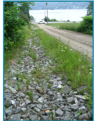
At left, lake association members seed and mulch a newly cleaned ditch. At right, a steep road that serves several camps has had a rock lining installed to prevent the previous on-going erosion of the ditch.
