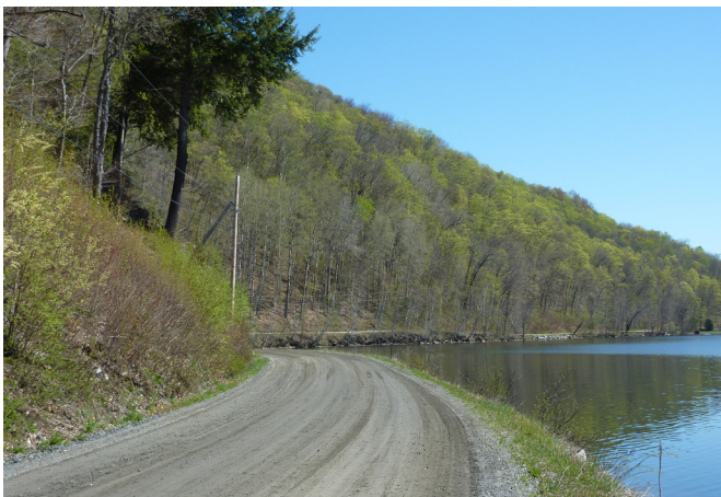
Proximity of this road to the lake combined with the narrow buffer zone contribute to risk of negative impact on water quality
